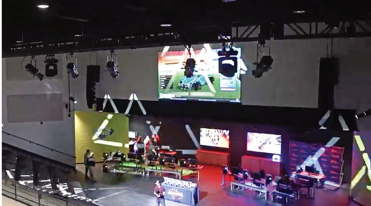
Two line array speaker systems, reinforced by more speakers and stage lighting on overhead rigging, pump-up the excitement. Animated pattern lights dance across the stage while gaming action appears on the videowall above the stage and on two on-stage displays.
