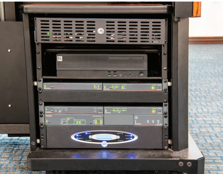
The NAV AVoIP products and other AV system components fit easily within the instructor station rack, occupying less space than the previous twisted pair AV switching system.
