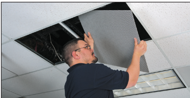
Installation in three easy steps: (1) Remove ceiling tile, (2) Make wiring connections, (3) Place speaker on grid and anchor with seismic tabs. Trim ceiling tile, if necessary, to fit with provided T-bar.
