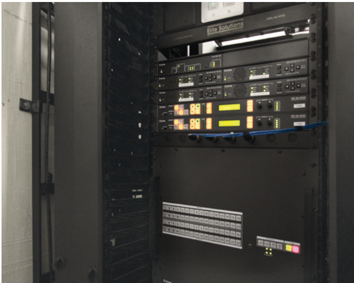
An equipment closet houses AV system central switching, scaling, streaming, and control equipment (Photo courtesy of Elite Solutions, Inc.).
