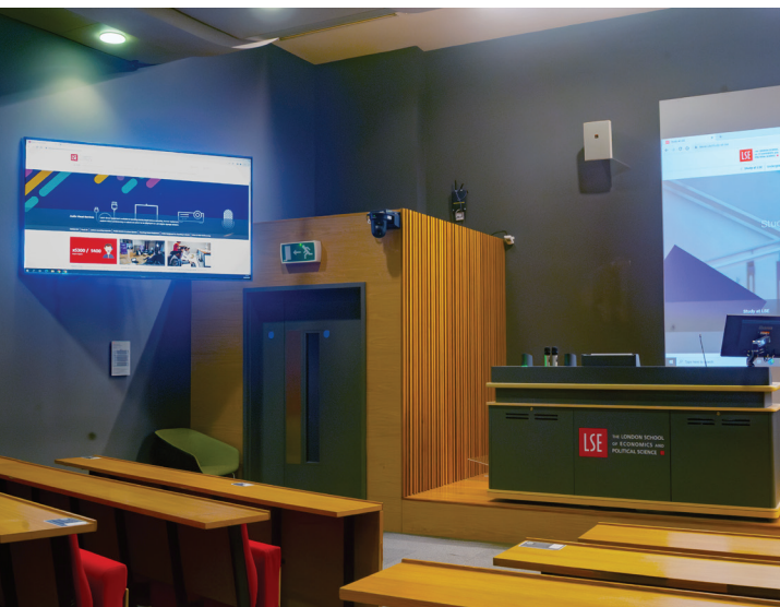
Stage-right flat-panel display provides presentation reinforcement, ensuring clear visibility for all attendees.
