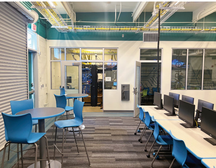
View looking into the IDF equipment room entrance.
