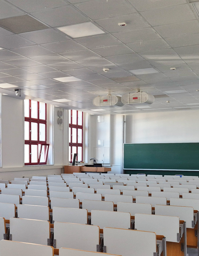
Lecture halls are equipped with primary and backup dual projectors, AV-equipped instructor desk, tracking PTZ camera, and ceiling array microphone. Small classrooms are equipped with a single projector, AV-equipped instructor desk, and ceiling-mounted speaker.
