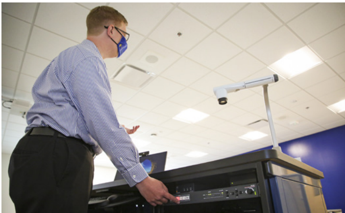
Instructors select AV content by simply pushing a button on the IN1606 switcher front panel. The switcher volume control knob adjusts sound level.
