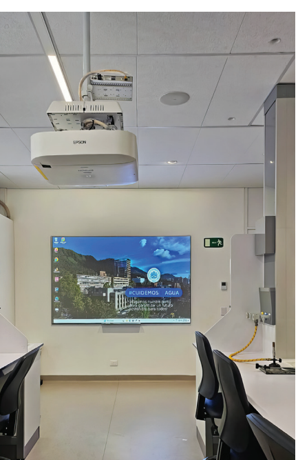
Typical laboratories are equipped with projectors, flat panel displays, PCs for sourcing AV content, and button panels that control AV system operation.
