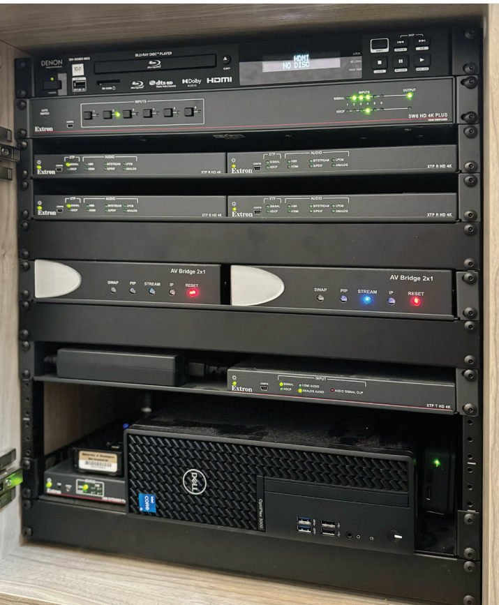
HIPs lectern AV equipment bay contains AV program content sources and switcher that selects which sources to send to the room's screens.
