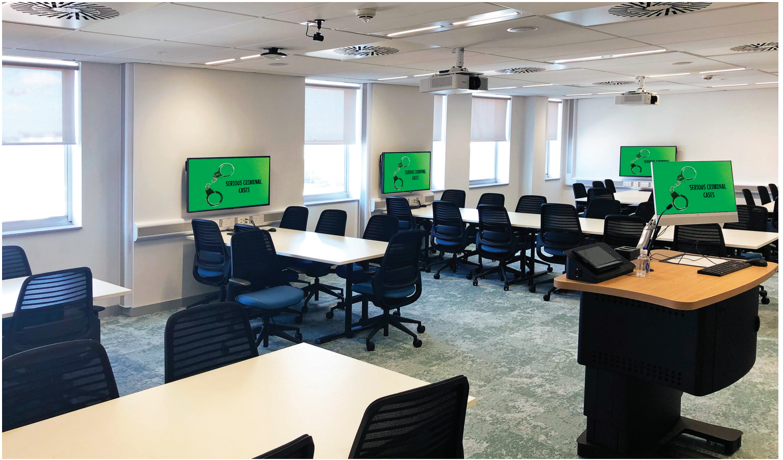
In UWE's collaborative learning spaces, the projection systems are fed by an Extron IN1608 xi scaling presentation switcher. The pod displays follow the main display until a student in that pod selects a different source. Sessions held in the interview rooms are shared live with the classrooms over the NAV® Pro AVoIP system.
